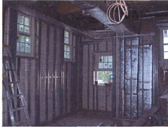
First Floor renovation
