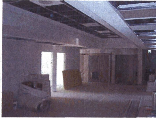
Second floor renovation
