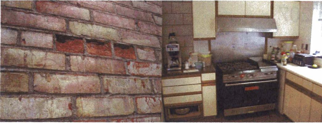
Spalling masonry
