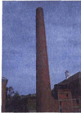
Large adjacent chimney
