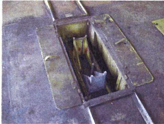
New lift equipment installation
