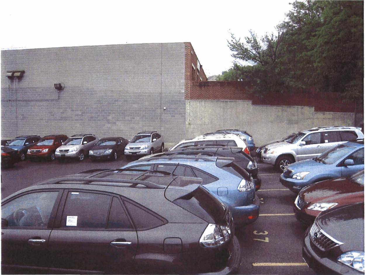
Figure 4: Commercial building, 3660 Wheeler Avenue
