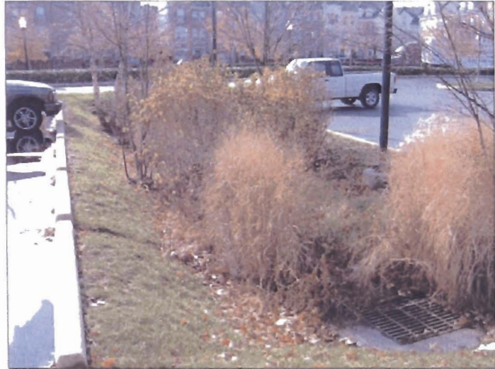
Figure 8-6. Bioretention Cells As Part Of Parking Lot Design. Beatley Central Library, Duke Street, City of Alexandria
