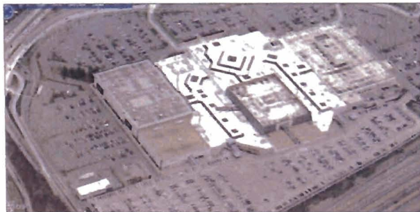
Landmark Mall. The large structure encloses an area as large as four to six typical city blocks.
