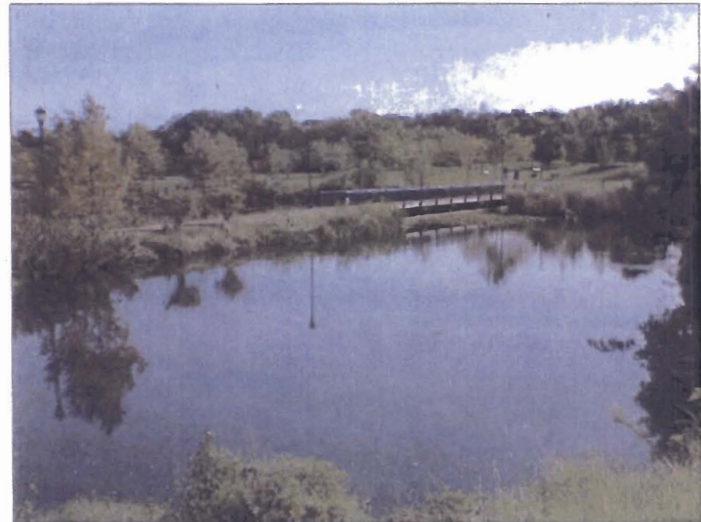
Figure 8-7 Stormwater Management Pond At Cameron Station. The Pond Located In Ben Brenman Park Collects Runoff From The Cameron Station Development Providing Both Stormwater Management And Aesthetic Benefits
