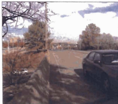
Pedestrians using the Van Dorn Street overcrossing of Duke Street must walk in the street.
