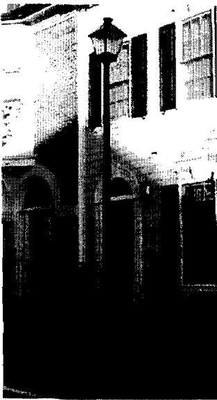
Dominion Virginia Power colonial light fixtures
