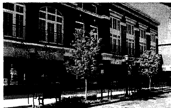
Mixed-use buildings should include a high-degree of transparency at ground floor commercial uses and a distinctly different façade treatment on upper residential floors, typically expressing bay dimensions of rooms and dwelling units. Examples shown here are in Atlanta.
