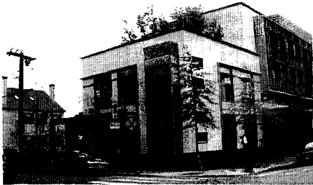
This building makes a transition to an adjacent residential street by terminating in a smaller building mass that matches the scale of nearby houses.
