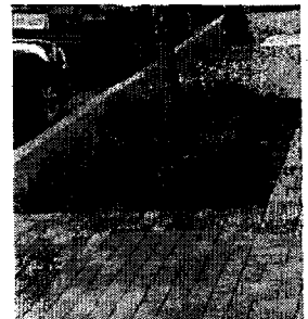
Tree wells should have contiguous tree trenches to encourage root growth and access to water, be flush with pavement, and be planted with groundcover.
