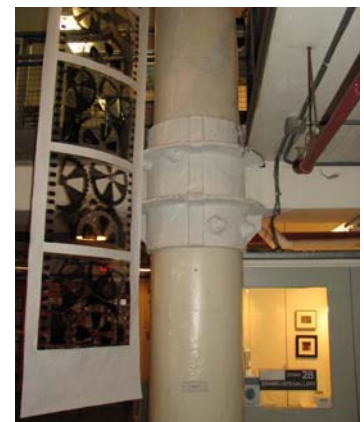
Column collars supporting the mezzanine level
