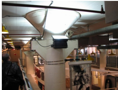
The mezzanine uses overhead lighting and indirect lighting located on support columns
