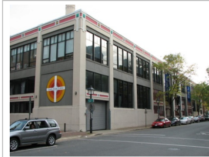
View of Torpedo Factory's northwest corner adjacent to Union Street
