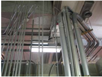
Conduits from the north utility room
