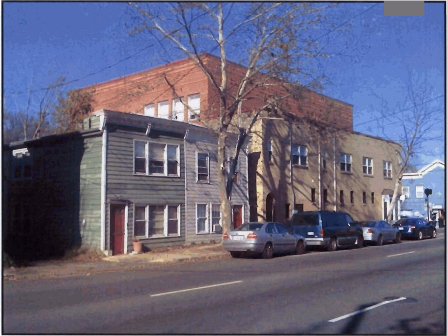
Figure 8: Photo of buildings across North Patrick Street.
