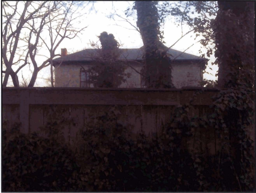
Figure 7: North elevation of house.
