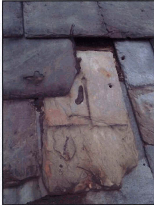
Figure 11: Photo of damaged slate.
