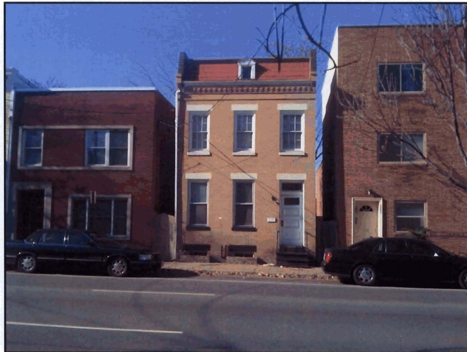
Figure 10: Photo of buildings across North Patrick Street.
