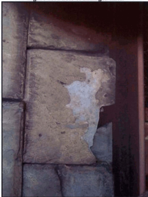
Figure 12: Photo of damaged slate.
