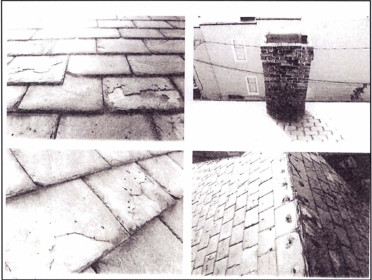
Figure 13: Photos of roof with damaged slate.
