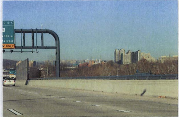
VIEW FROM WILSON BRIDGE LOOKING WEST
