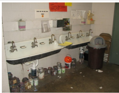
Mezzanine clean up sinks have sediment traps
