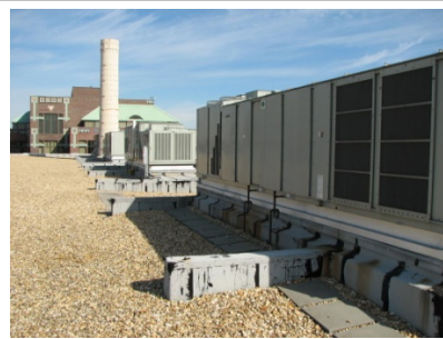
Four HVAC units are located on the roof along the building's north-south centerline
