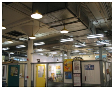
Ductwork is exposed and suspended from each floor's ceiling
