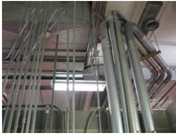
Conduits from the north utility room
