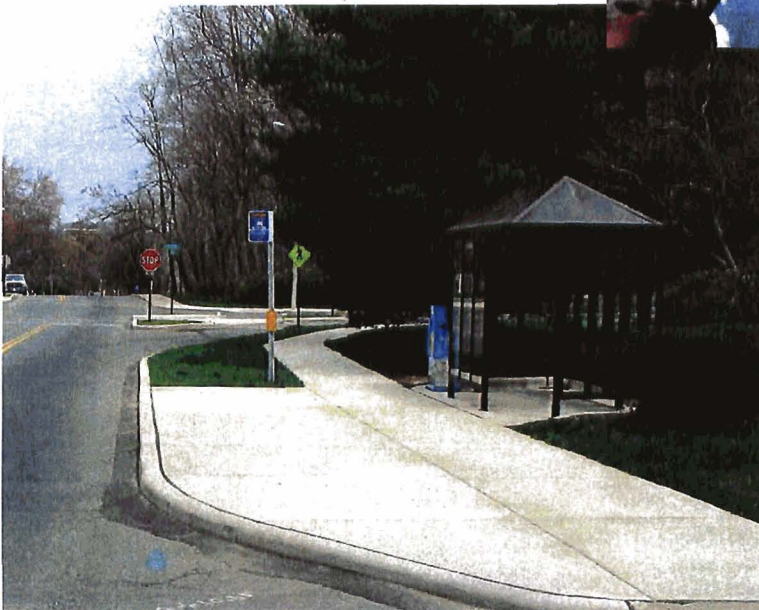
Bus Pad and Bus Shelter on Valley Drive in Alexandria
