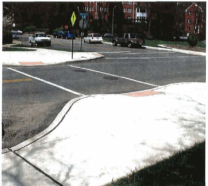
Unsignalized street crossing with sidewalks, marked crosswalk, accessible curb ramps, and curb extensions on Valley Drive
