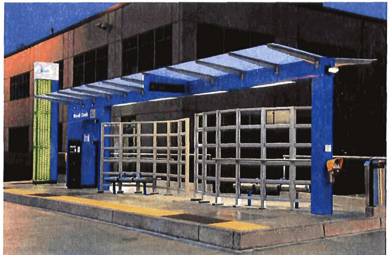
Swift bus station in Washington State with seating, shelter, information kiosk, and ticket vending machines
