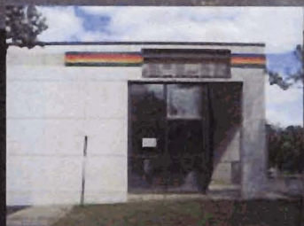
WEST CORNER AT BUILDING ENTRY
