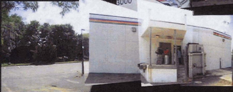
EAST BUILDING ELEVATION AT LOADING DOCK
