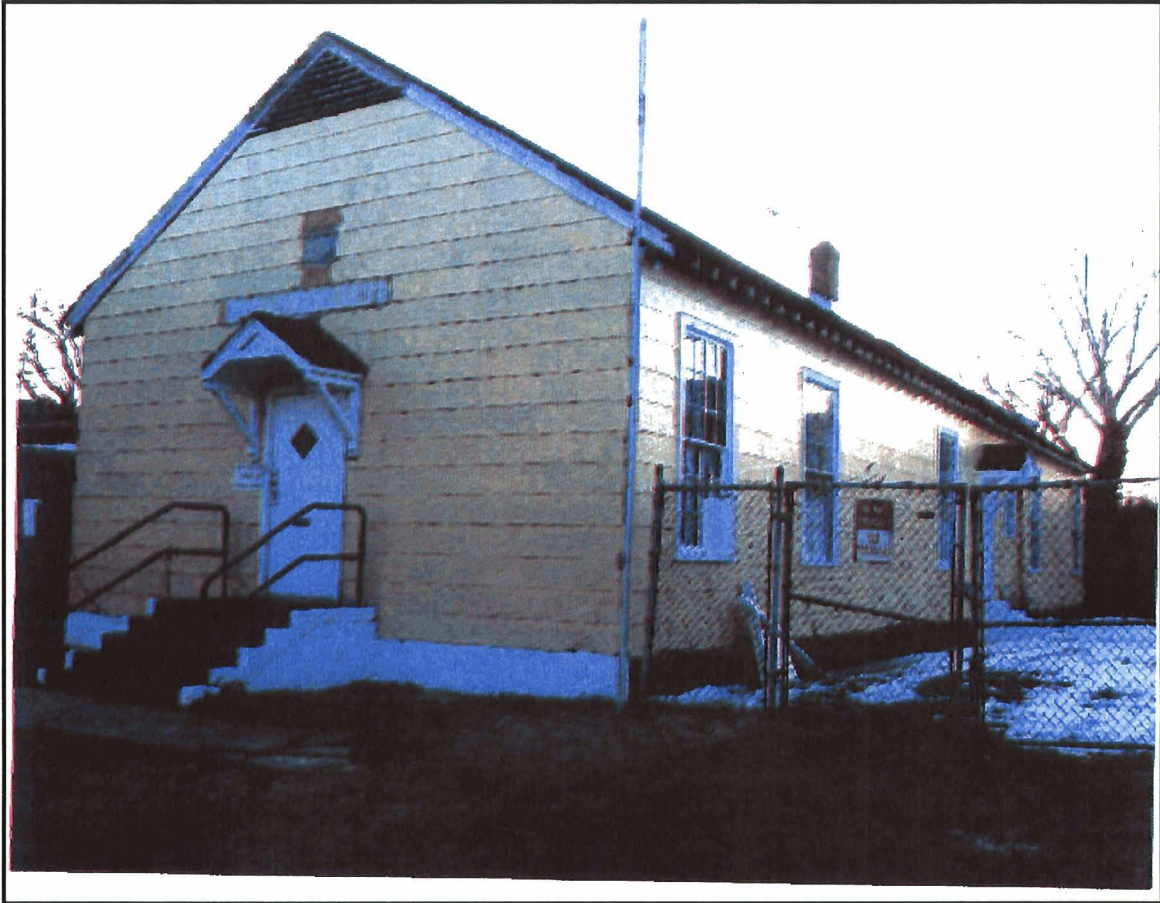
Figure 2. Existing exterior condition photograph from N. Fayette Street.
