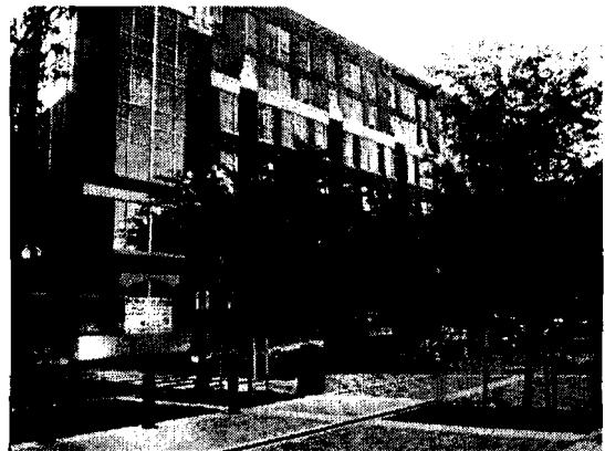
333 John Carlyle Street mixed-use building showing vacant southeast corner of ground floor.
