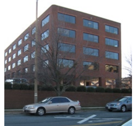
Existing Pipefitters Union Building
