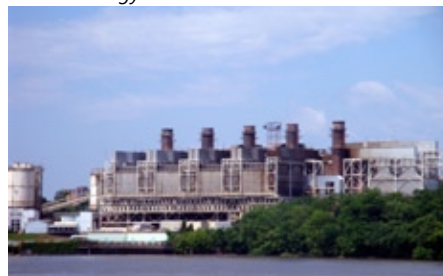
GenOn Energy Power Plant
