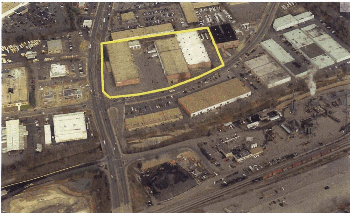
View of Landmark Gateway site looking north
