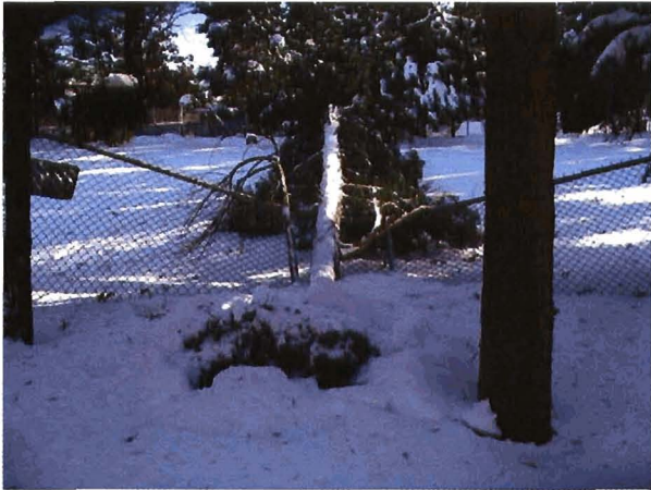
City tree damage to OBC Cemetery fence Photo: G. Eugster
