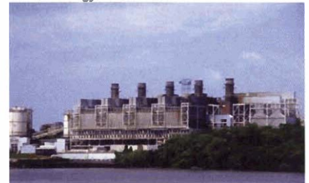
GenOn Energy Power Plant
