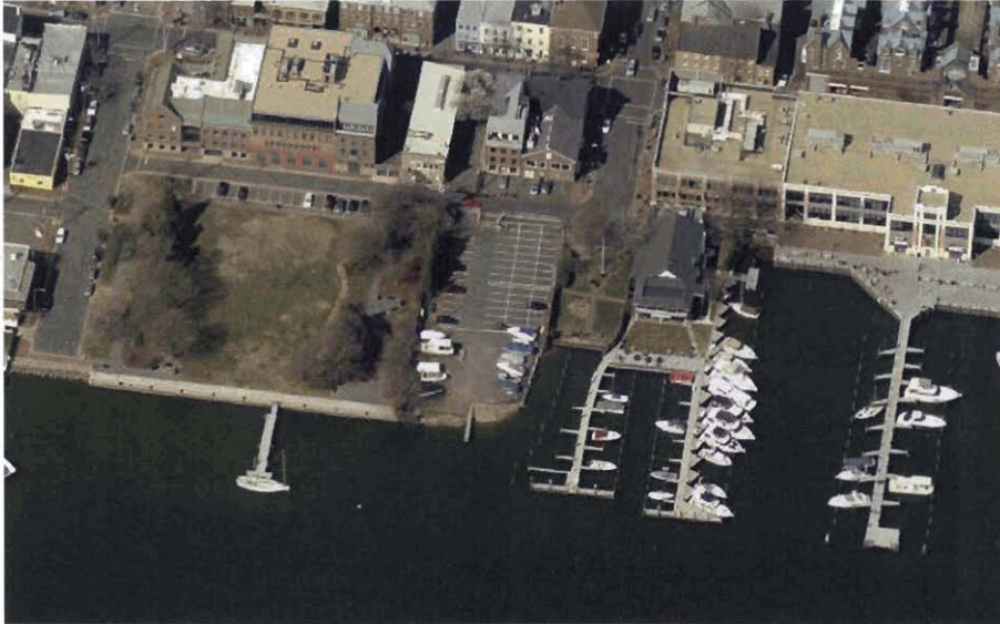
Aerial view of existing condition at the foot of King Street
