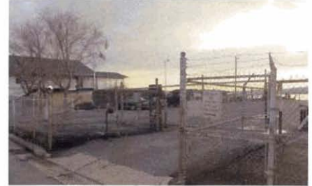
Existing ODBC Parking Lot
