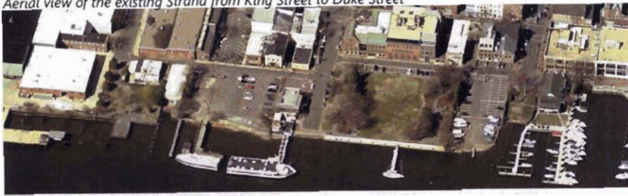
Aerial view of the existing Strand from King Street to Duke Street
