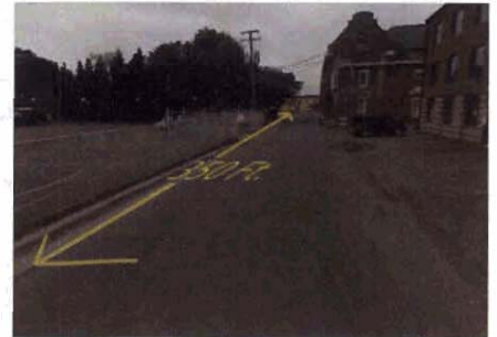
Looking South on The Strand past what is currently an Inactive Frontage
