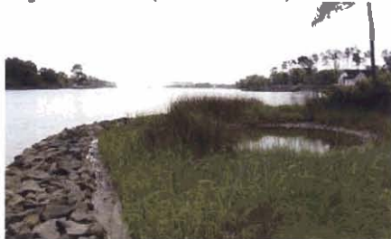
Structural Revetment for Shoreline Naturalization (Center for Coastal Resources Management, Virginia Institute of Marina Science)
