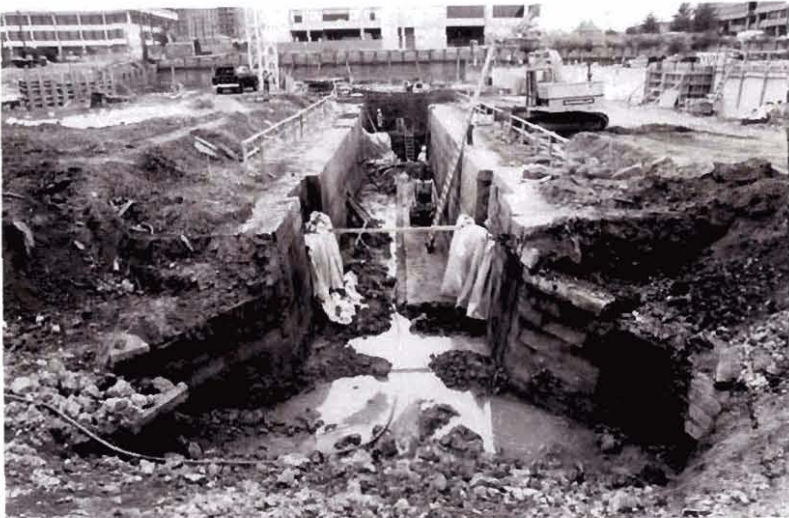
Excavation and restoration of the Tide Lock of the Alexandria Canal in Alexandria
