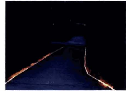
Lighting imbedded in pavement
