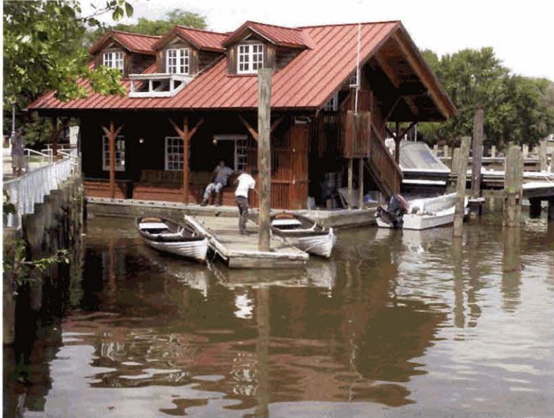
Floating office and workshop of the Alexandria Seaport Foundation, City Marina
