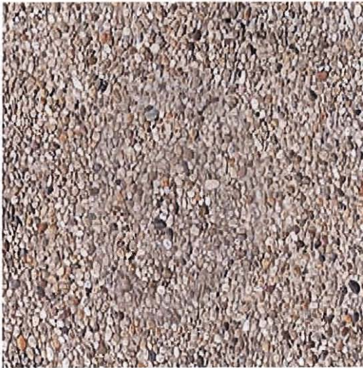
Exposed aggregate concrete
