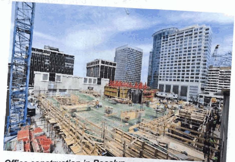
Office construction in Rosslyn
