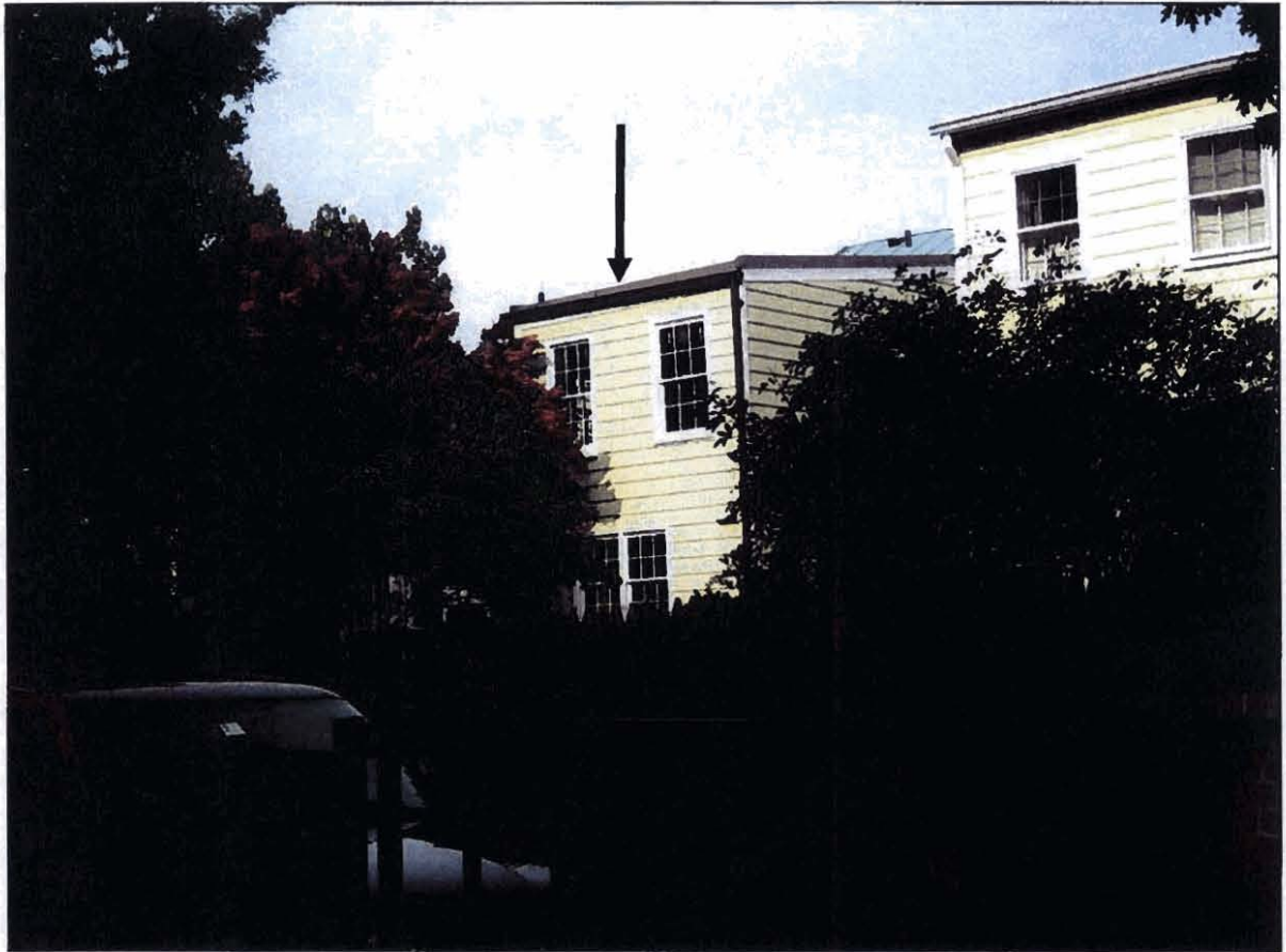
Figure 3: East (rear) elevation as viewed from Princess Street.
