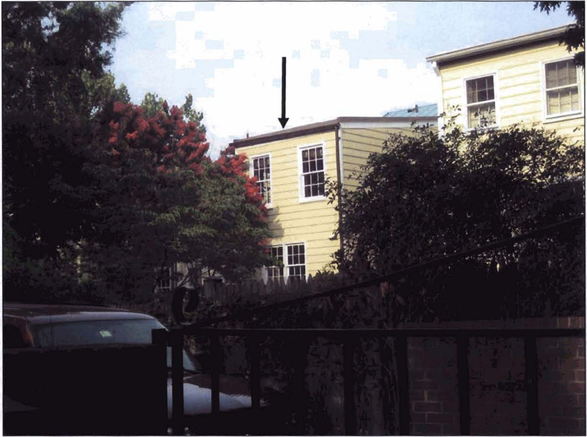
Figure 5: East (rear) elevation as viewed from Princess Street.
