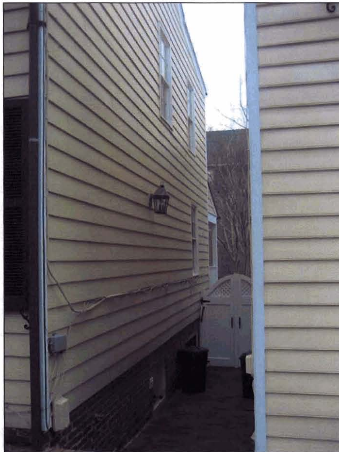
Figure 4: South (side) elevation and shared alley showing the existing open porch in the rear.
