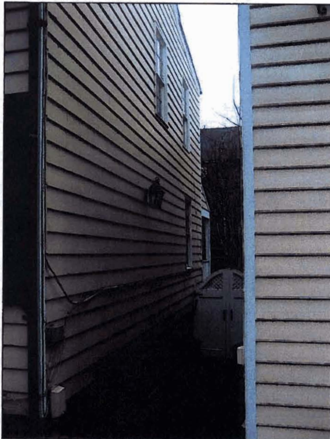
Figure 2: South (side) elevation and shared alley showing the existing open porch in the rear.
