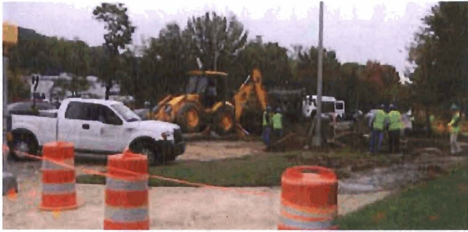
The intersection of Walter Reed and Arlington Mill on October 11, where WSS emergency crews worked to repair a broken water main. Photograph by Gretchen Fallon.
