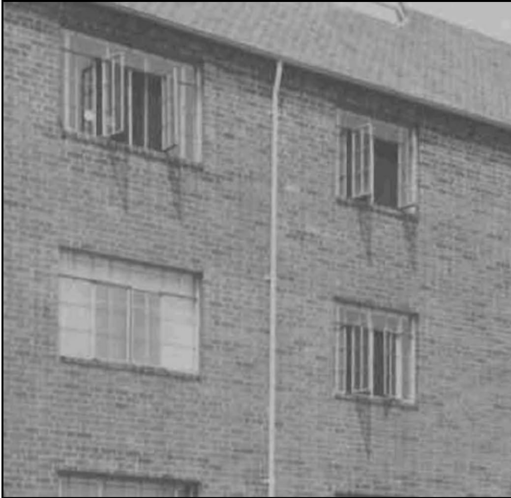
Figure 6. Detail of historic photograph, circa 1942
