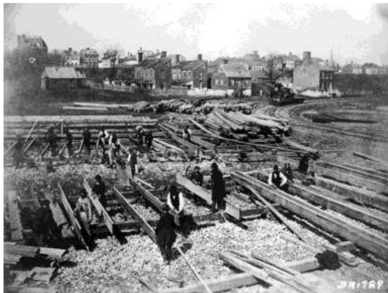
Workers of the USMRR probably assembling bridge trusses at the foot of Franklin Street, ca. 1863 Library of Congress
