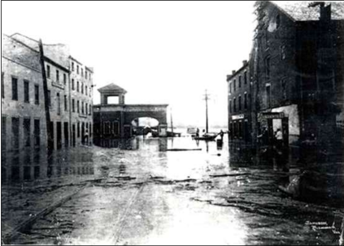
Foot of King Street showing arch of ferry building, 1900. Alexandria Library-Local History/William F. Smith Collection
