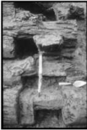
18th Century Wharf Bulkheads
