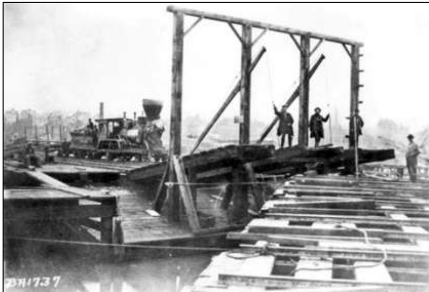
The innovative USMRR transfer bridges for loading barges with railcars, Franklin Street. Library of Congress
