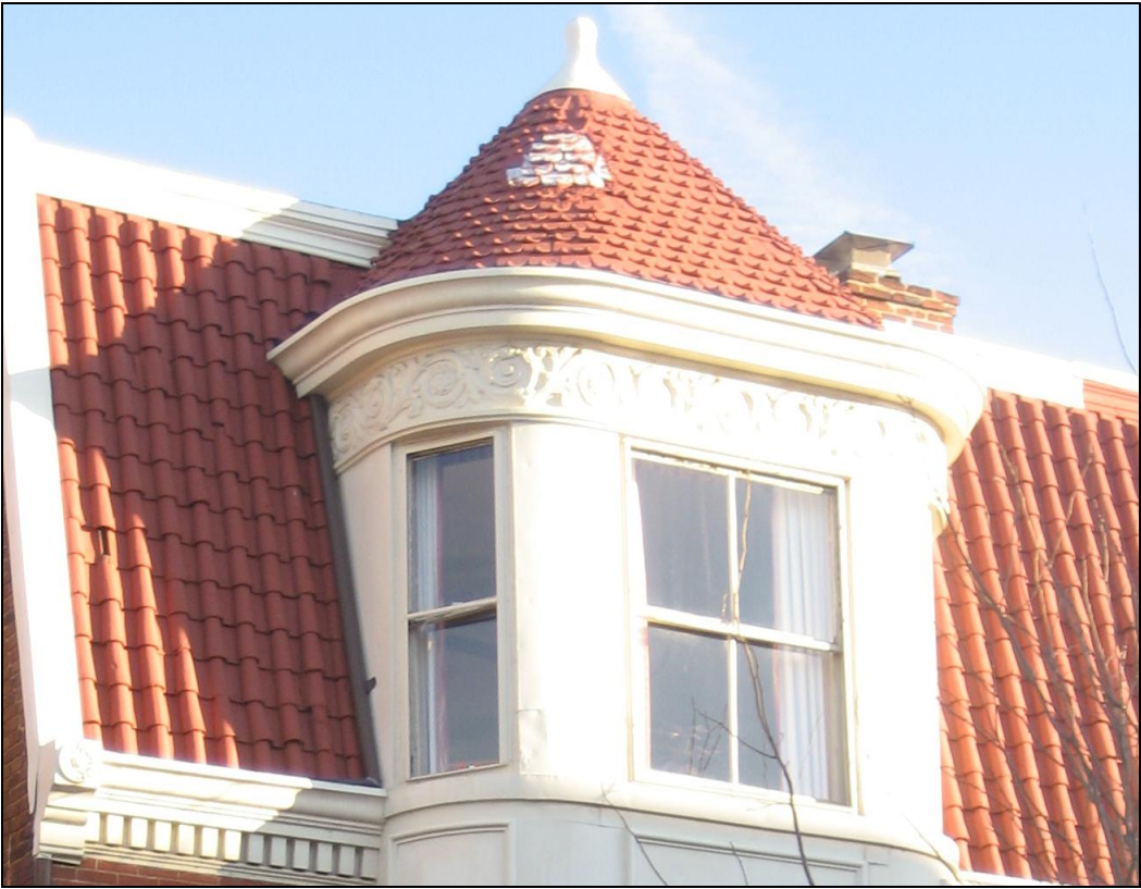
Figure 2. Detail of existing roof material on turret and mansard.
