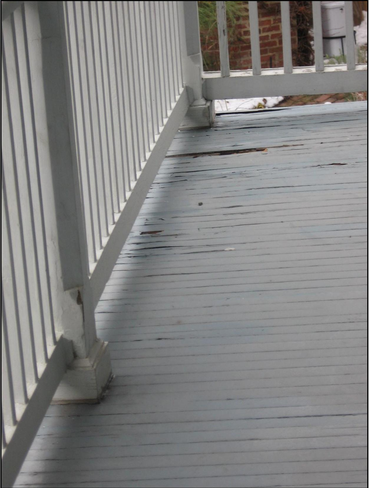
**Figure 3. Photo of porch floor damage.**
