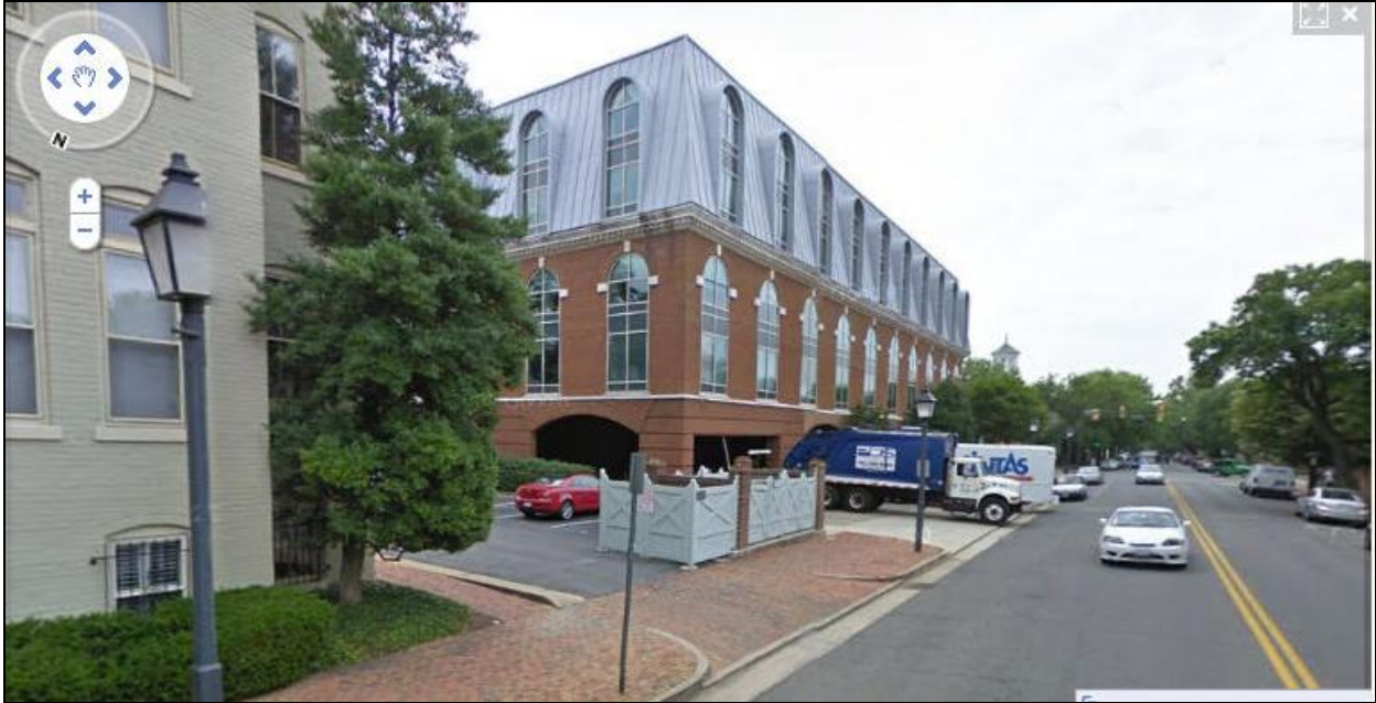
Figure 2. View of existing enclosure and Atrium Building, looking south on South Columbus Street.
