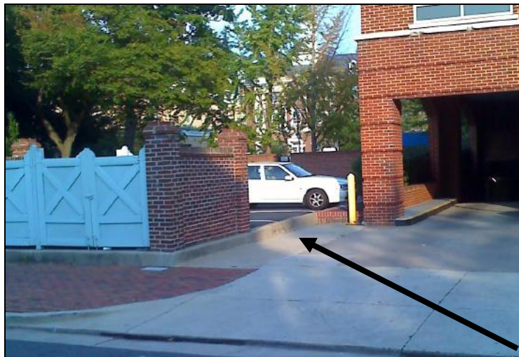
Figure 3. Existing utility enclosure and area of expansion, looking east.
