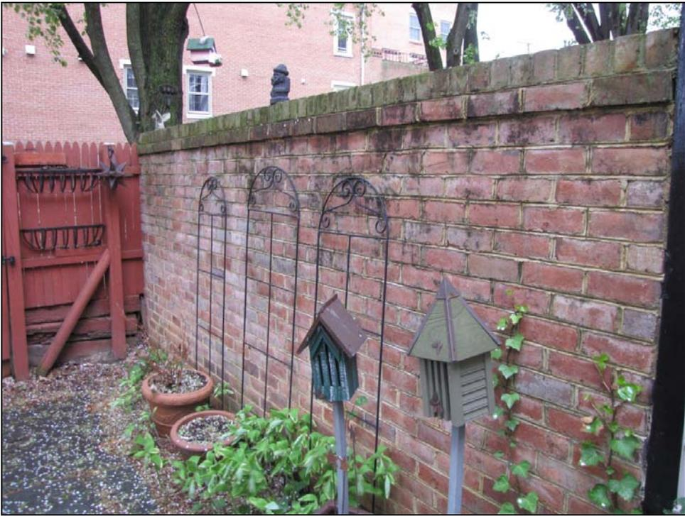
**Figure 5: Brick wall between 716 and 718 Gibbon. Proposed wall will match both the dimensions and color of the existing neighbor's wall.**
