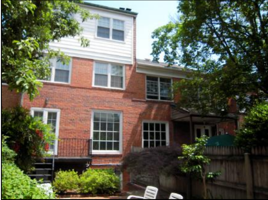
Figure 5. Rear façade of 821 S Lee Street (left) and 823 S Lee Street (right).
