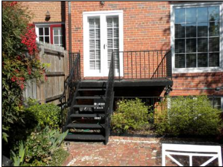
Figure 1. Existing rear iron deck at 821 S Lee Street to be removed.
