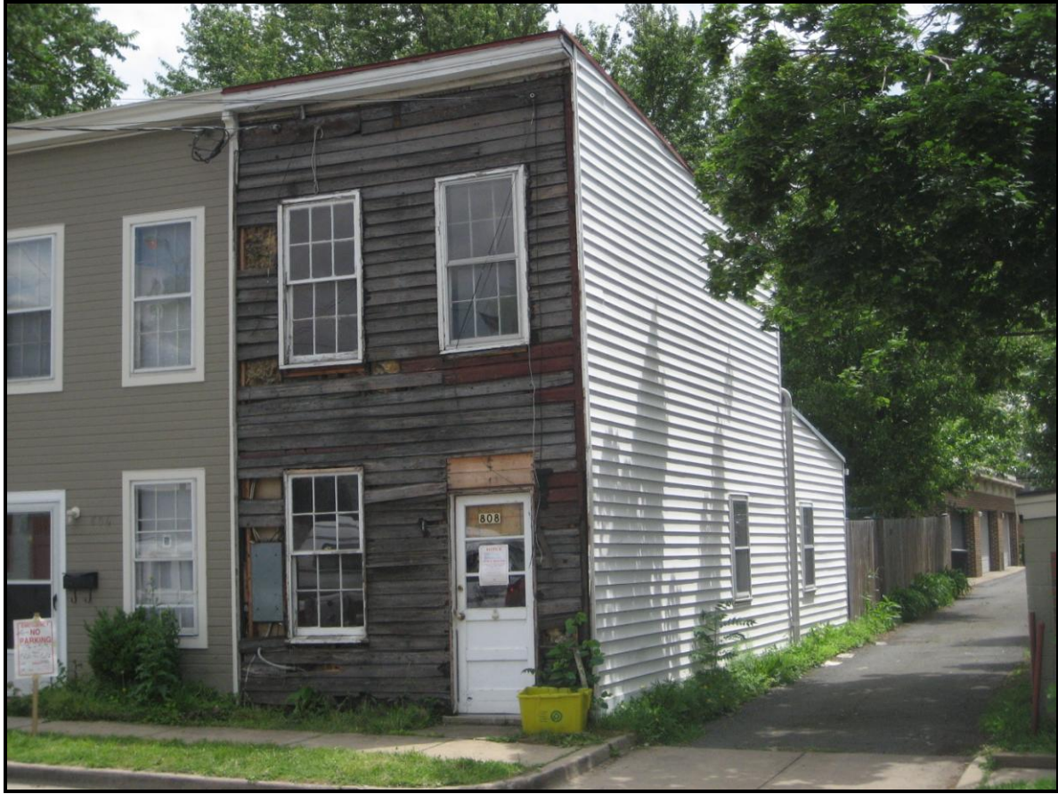
Figure 2: Photo of 808 Pendleton Street taken on May 19 th , 2011 showing the front façade after the removal of siding and bricktex.
