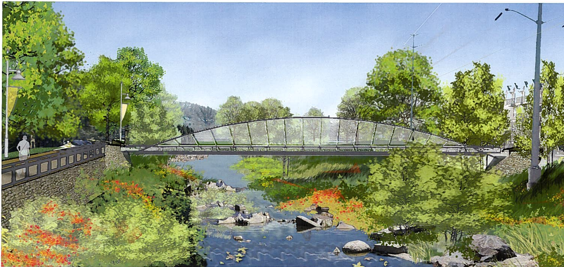
PREFERRED CHANNEL CROSSING DESIGN: Open span design allows unimpeded storm flow and wildlife movement.
