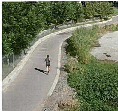
Asphalt trail with infiltration strip
