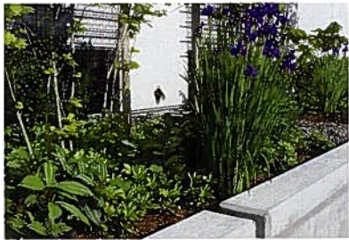
Stormwater planter with slotted curb
