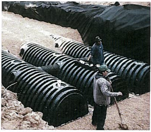
Proprietary underground storage device (manufactured by StormChamber), detail/section above, photo left
