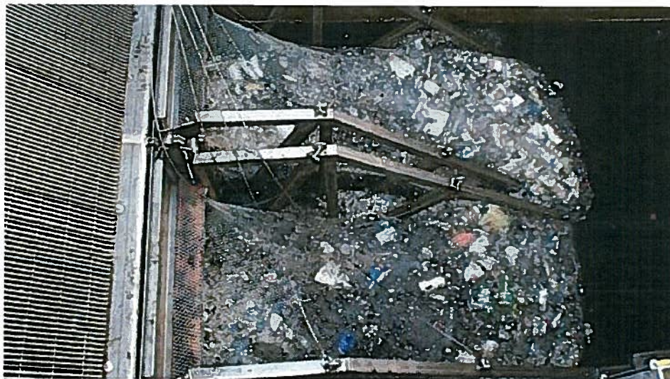
Example of a custom fabricated litter interceptor, detail/section above, photo below
