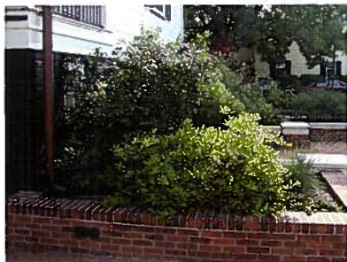
Stormwater planter connected to roof downspout
