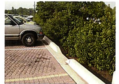
Parking that incorporates permeable paving or other LID stormwater management technology can mitigate the impact on Four Mile Run.
