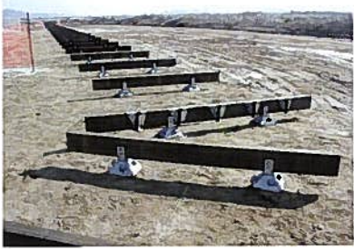
A boardwalk support structure designed to minimize disturbance
