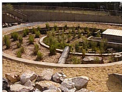
Stormwater planter connected to roof downspout
