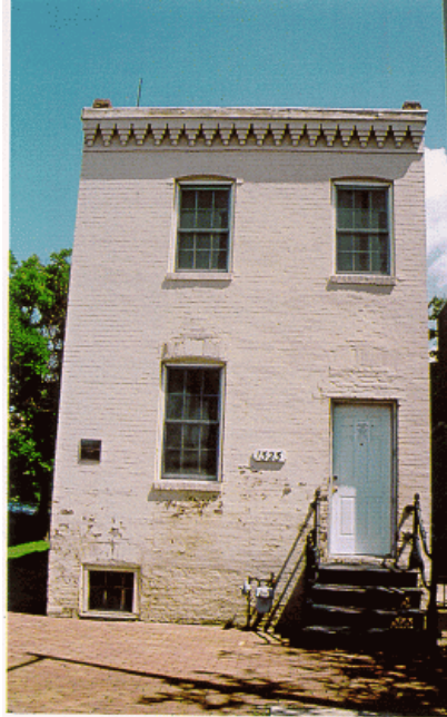
Current condition photograph of 1323 Duke Street
