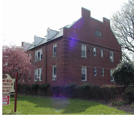
Figure 3 Gunston Hall Apartments, designed in a conscious Colonial Revival style in 1939, employs many of the same design elements as the original Gunston Hall plantation building including brick construction, slate covered gable roof with dormers, double chimneys, pedimented door surrounds quoining and circular windows.
