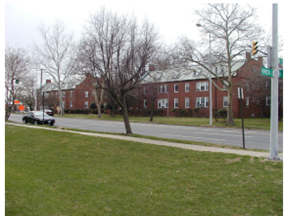
Existing Gunston Hall Apartments
