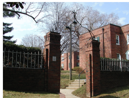
Figure 9 Colonial Village courtyard entrance.
