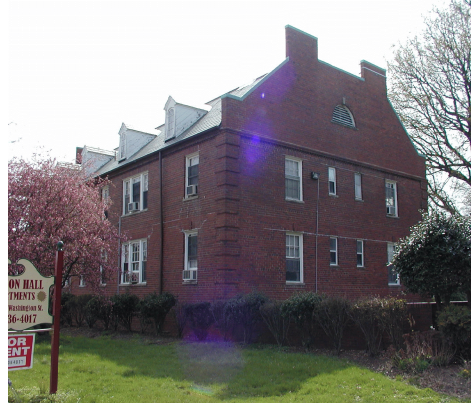
Figure 6 Gunston Hall Apartments, designed in a conscious Colonial Revival style in 1939, employs many of the same design elements as the original Gunston Hall plantation building including brick construction, slate covered gable roof with dormers, double chimneys, pedimented door surrounds quoining and circular windows.
