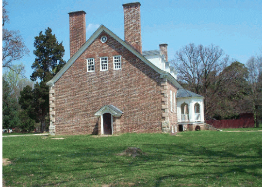
Figure 5 Gunston Hall, home of George Mason, Mason Neck, Virginia. Constructed 1755-60.
