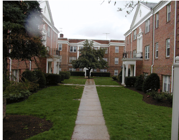
Example of Typical Garden Apartment Scale and Mass
