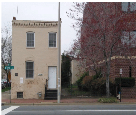
Current Condition Photograph of 1323 Duke Street
