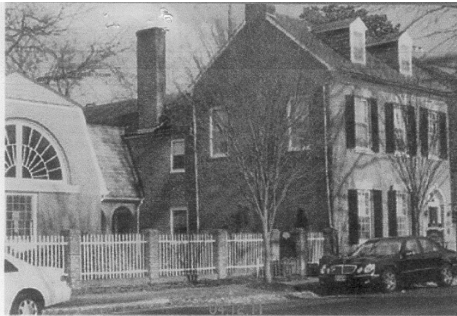
Figure 1 - Front elevation with two part addition to left
