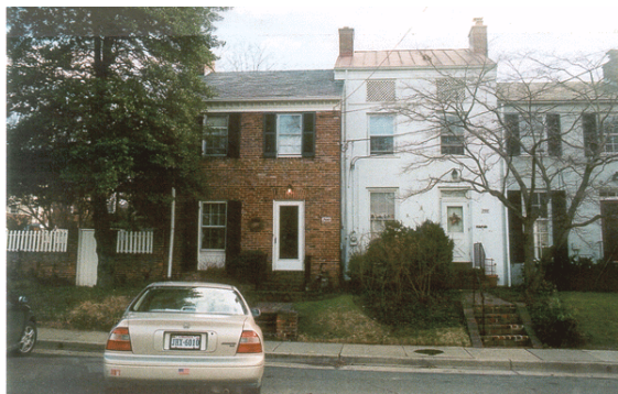
Figure 1 Front (west) elevation
