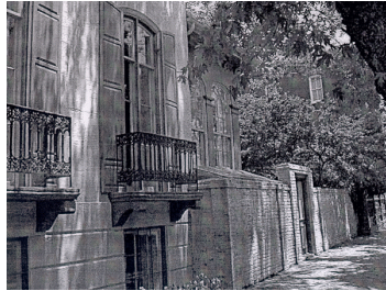
Figure 2 Garden wall facing Prince Street
