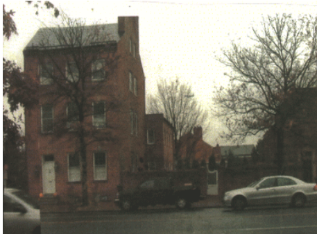
Figure 1 View from North Washington St
