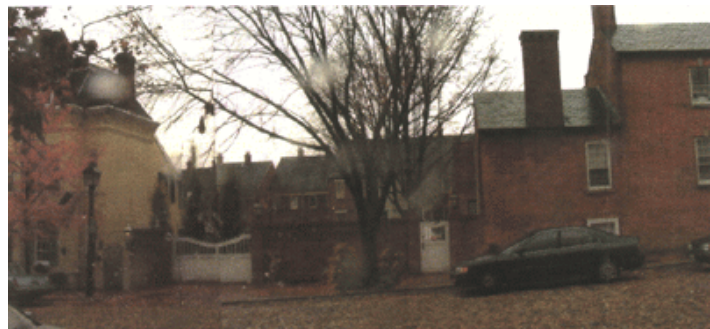
Figure 2 View from Princess St
