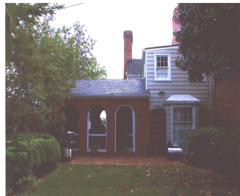
Figure 2: Existing rear view
