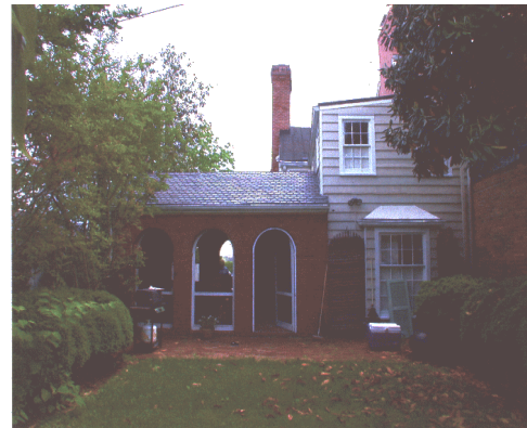
Figure 2: Existing rear view
