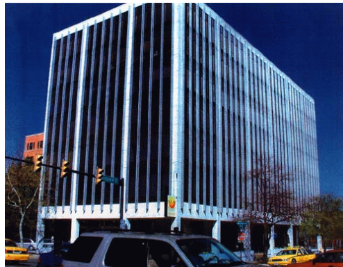
Figure 1 Existing Jefferson Building at 901 North Washington St
