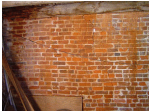
Figure 2 Lower portion of existing interior south wall
