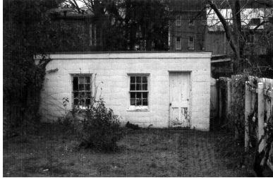
Figure 4 - yard side of garage
