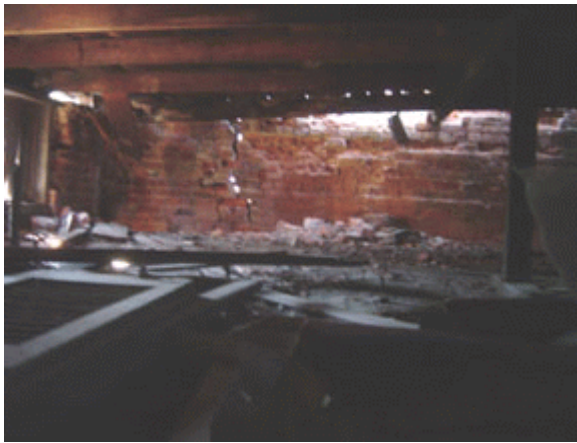
Figure 1 Upper portion of existing interior south wall
