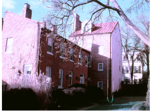
Figure 1 South (rear) and East (side) elevations
