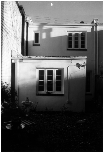
Figure 1 - One story rear ell to be demolished
