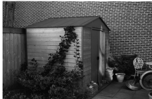
Figure 2 - Shed to be removed
